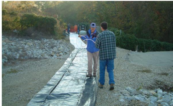
Figure 6-2 Tubing Being Pulled to Reference Mark
