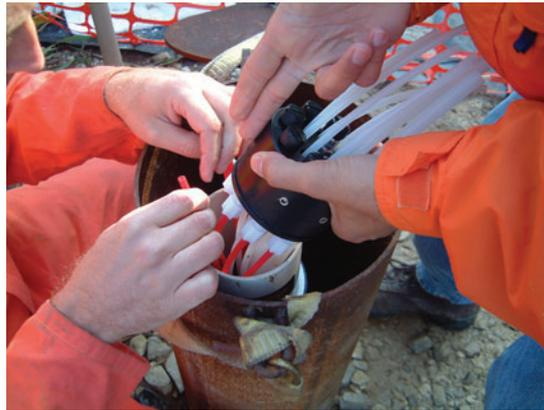
Figure 9-3 Pump Tubing Being Attached to a Wellhead
