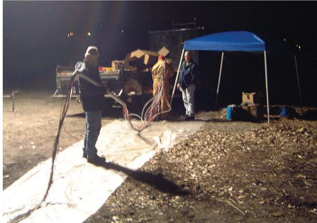
Figure 4-5 Casing Section Being Threaded Over Monitoring Tubing
