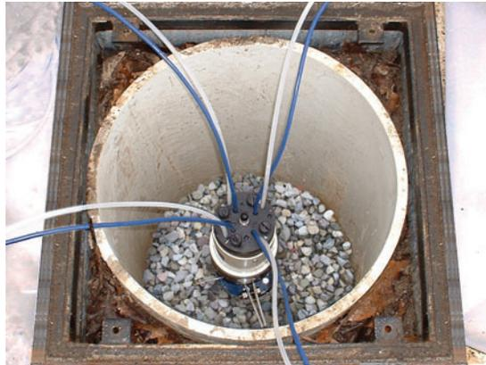
Figure 9-1 Tubing Organized Around the Wellhead
