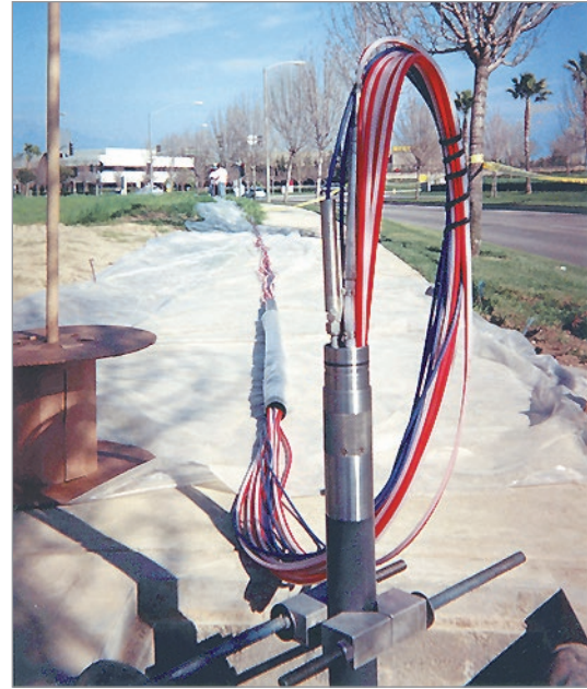
Contaminant investigation at a U.S. Air Force Base. Waterloo Systems installed to 700 ft. in overburden using screened and cased wells. Up to 6 zones per hole with dedicated pumps and transducers.
