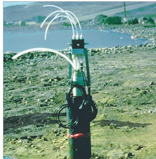
Landfill site over fractured granite, monitored with five Waterloo Systems. Each System comprised of dedicated Double Valve Pumps and Pressure Transducers in 4-6 intervals to depths of 275 feet (84 m). The Multi-Purge Manifold allowed the monitoring of 21 zones to be completed in less than 2 days.
