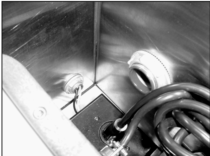
Figure 1-10 Detail of cabinet interior showing the plug-in for the power pack
