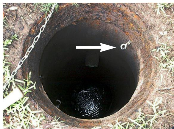
**Figure 5: Eyebolt suspension in manhole**
