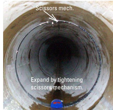
**Figure 25: Expand and secure the ring against the channel wall**
