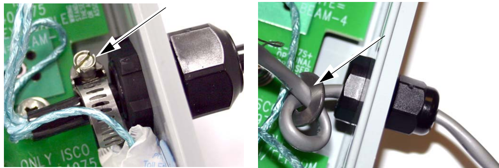
Figure 3-10 Strain relief for sensor extension cables
