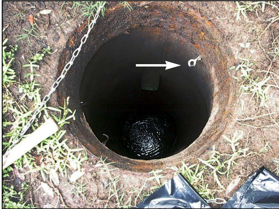
Figure 2-34 Lag shield - eyebolt manhole mounting
