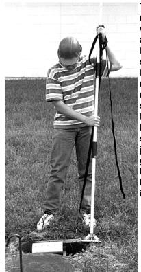
This picture shows the correct position of the installer when placing the device in a manhole. He is standing fully upright and off to one side of the manhole. His feet are set apart to help maintain balance and he is not leaning on the pole for support. In this stable position he is unlikely to slip or lose balance even if a strong current in the sewer jerks the pole from his grasp. Because he is not leaning over the manhole, he is in little danger of falling in.
