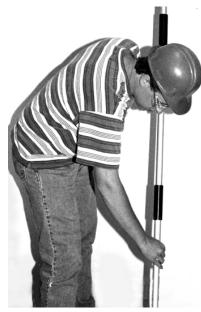
In this picture, the installer has gripped the pole too far down. This forces him to bend at the waist, and puts his upper body directly over the manhole. In this dangerous position he is actually depending on the pole to help maintain balance. If the force of the flow stream were suddenly to jerk the pole sharply or pull it from his hands, he could easily lose balance and fall into the manhole.
