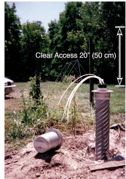
Figure 9-6 Above ground completion Minimum 6" dia. (15 cm) and 20"(50 cm) clearance is required
