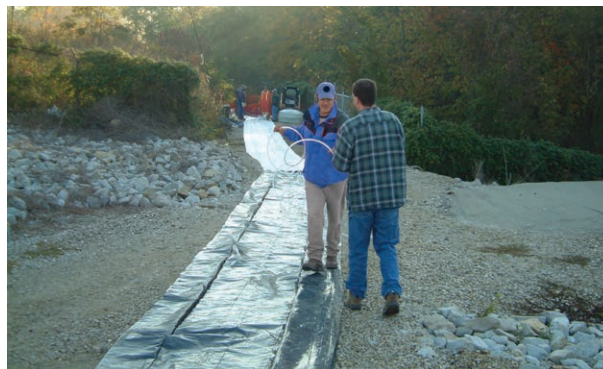
Figure 6-2 Tubing Being Pulled to Reference Mark
