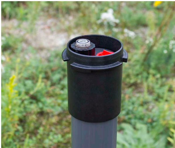
Remove Existing Levellogger Installation
