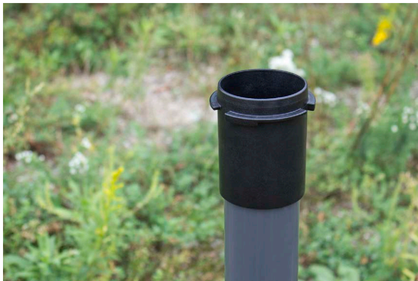
Figure 6-3 Install the Well Cap Base
