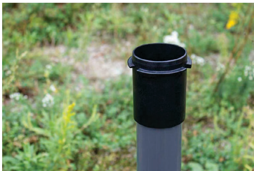
Figure 6-3 Install the Well Cap Base
