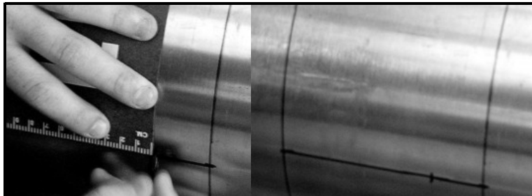
Figure 28: Measuring and Marking Spacing
