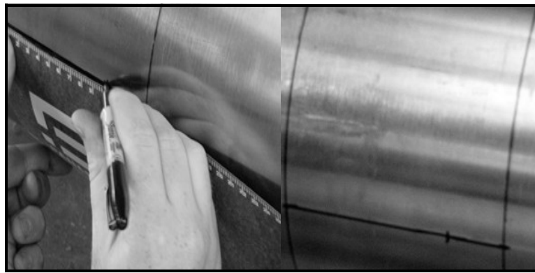
Figure 24: Marking the 9 o'Clock Position
