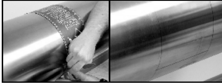
Figure 23: Marking the 3 o'Clock Position
