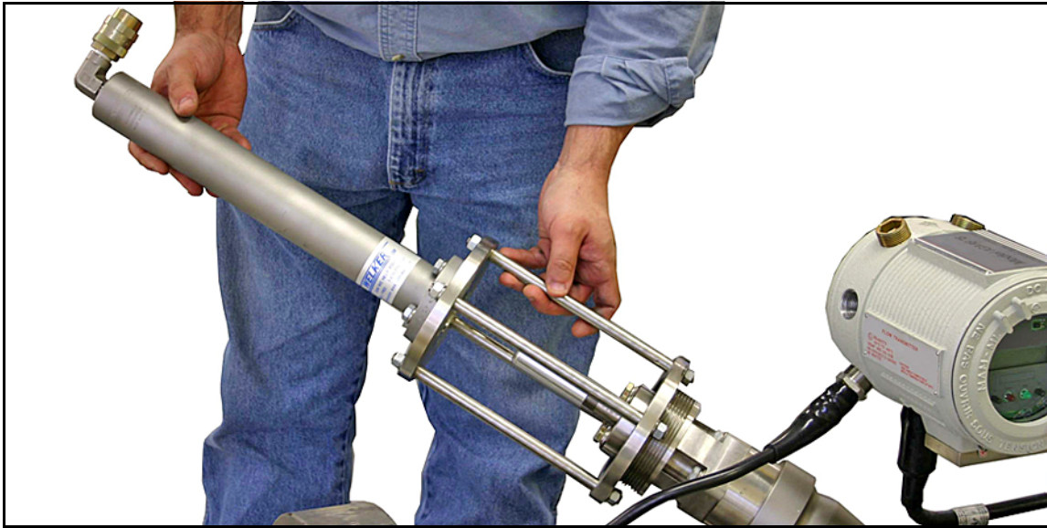
Figure 7: Installing the Insertion Mechanism
