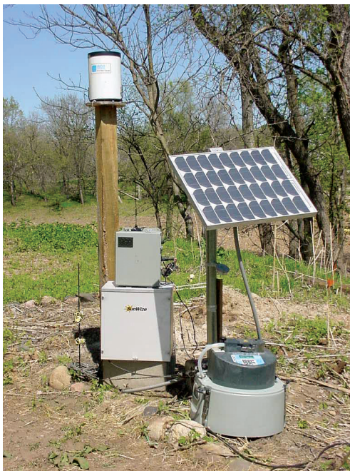
A 674 rain gauge connected to a Teledyne ISCO 6712 or Avalanche sampler is ideal for collecting rainfall data as well as runoff-triggered samples at remote monitoring sites.
