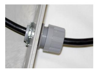
Figure 2-10 Position and secure the cable
